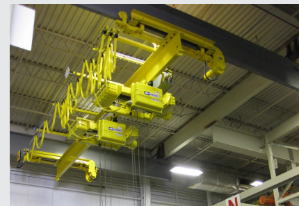
Louden crane with Speedway hoists.
